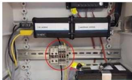
Figure 8d: Pipe & Reference IN
